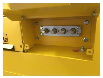
Connect the cable to above three phase and four wires terminals.
